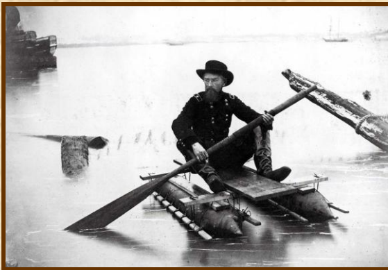
Union General Herman Haupt, a civil engineer, moves across the Potomac River in a one-man pontoon boat that he invented for scouting and bridge inspection.
